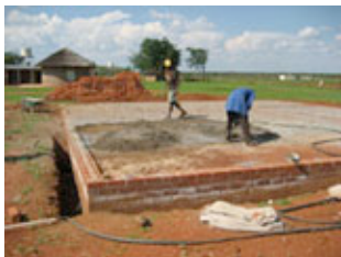
Foundation of the Fulleton/Reyman Memorial Guest house at KCV
