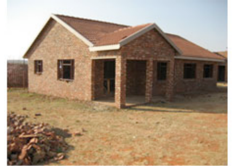
Minister's house at Tigane which is also used as the church
