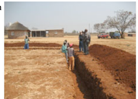
Foundations begun for the Fulleton/Reyman Memorial Guest House
