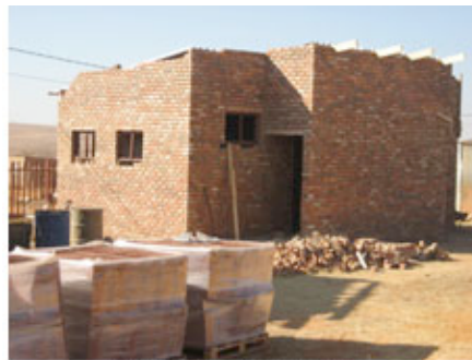
Tigane-Toilet block, roof nearly finished
